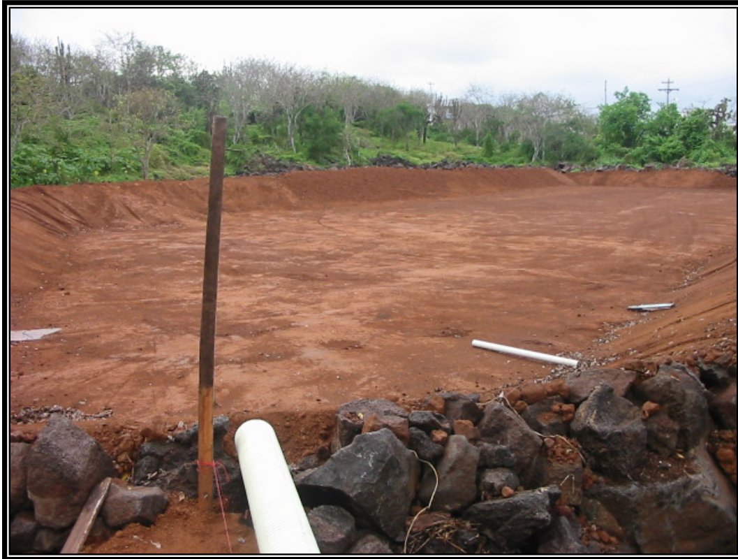
Figure 6. Finished platform for Artificial Wetland, Puerta Ayora, Galapagos Islands.
