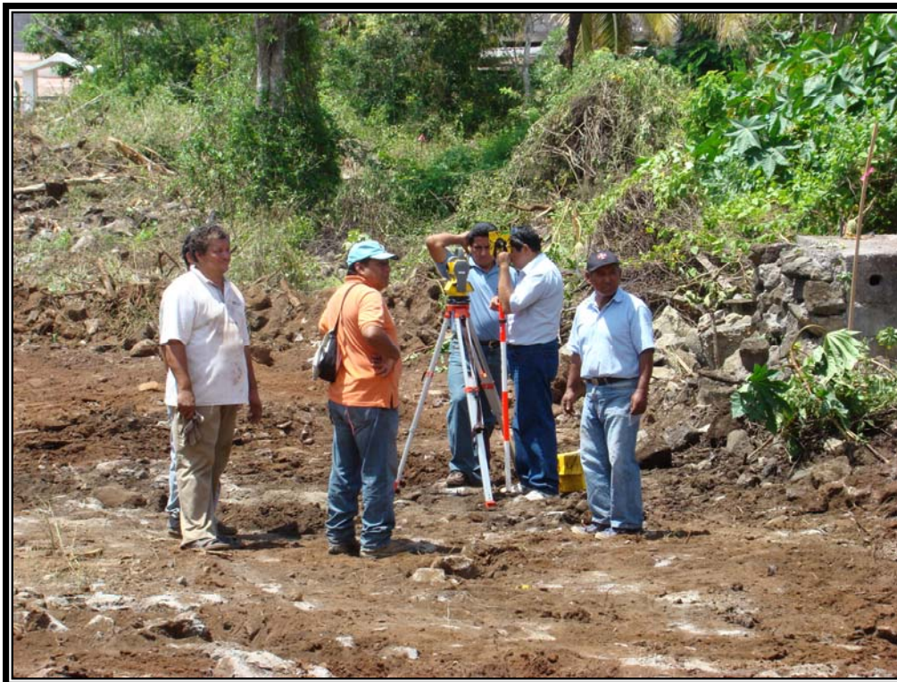
Figure 5. Engineers and workers survey the construction site.
