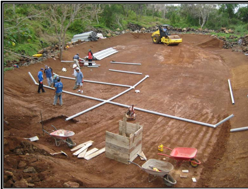
Figure 7. Pipe laying in the Artificial Wetland cell, Puerta Ayora.
