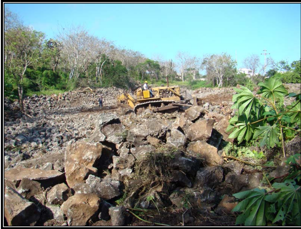
Figure 4. Early Construcion on the Artificial Wetland System for Puerta Ayora.
